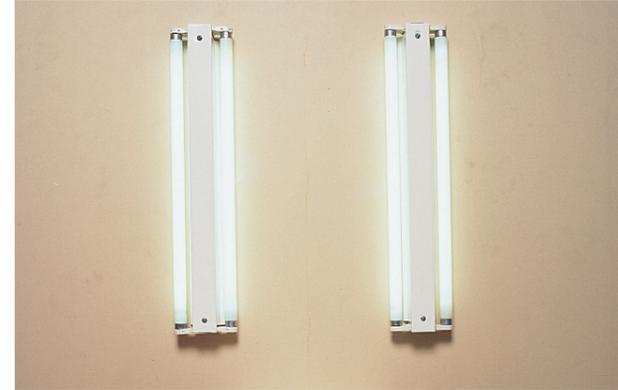
In some circumstances, fluorescent lights installed directly over butt joints may help to conceal the joints
