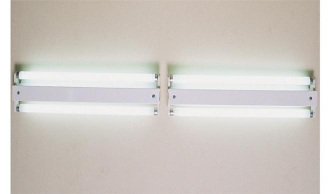
Fluorescent light tubes should not be run parallel to the long edges of plasterboard sheets
