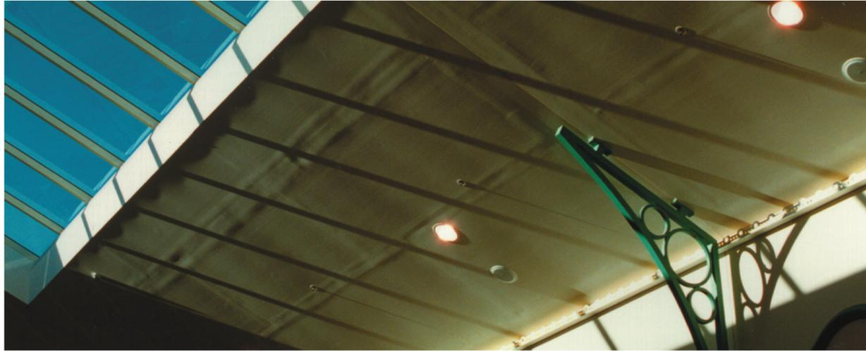
A plasterboard ceiling under glancing light conditions
