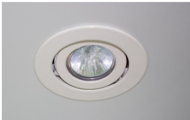
Recessed downlights and spotlights avoid glancing light by providing an even downward illumination
