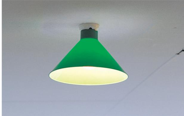
An opaque shade directs the light downwards to illuminate the room not the ceiling
